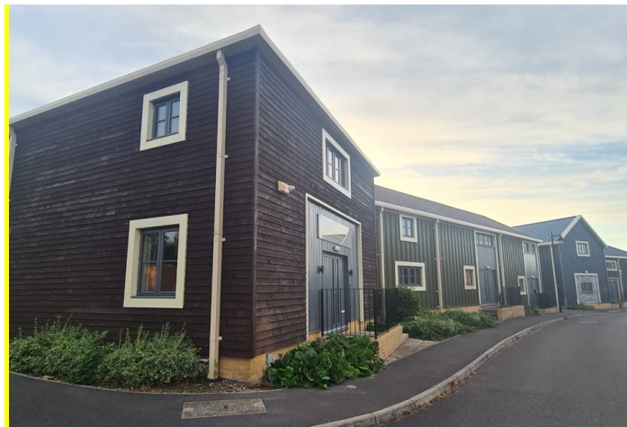
Light industrial and commercial buildings in a mixed-use development with windows and doors fronting onto the street creating 'active frontage' and a built form which is in keeping with residential form, Tisbury, Wiltshire. (Credit: Create Streets)
