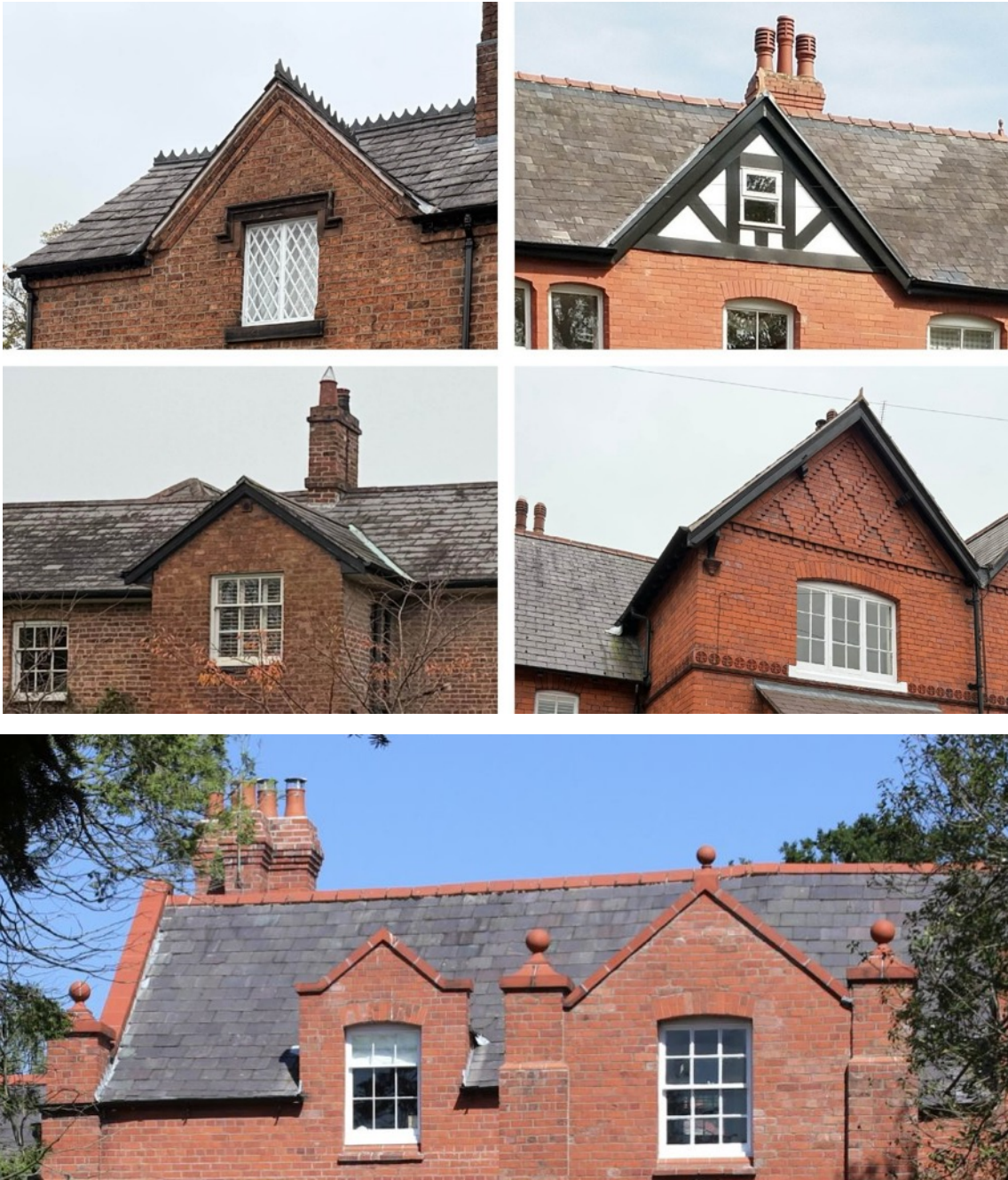
Examples of local roof material. Note the detail brick and timber work of the gables.
