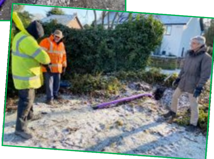
Cable pulled in and now waiting for BT
