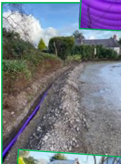
The trench in the car park
